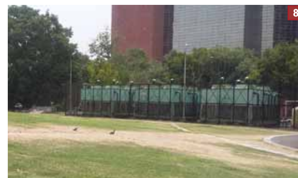
Air Conditioning Plants and Cooling Water Tank
