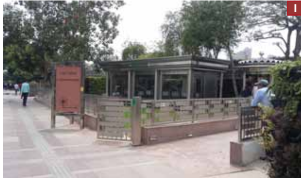
Weaver's enclosure and ticket counter; at footpath level
