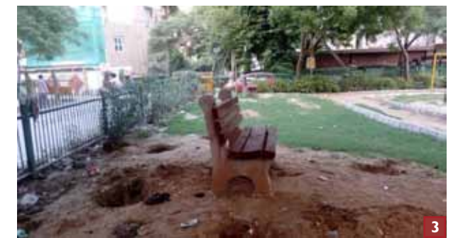
Lack of maintenance
