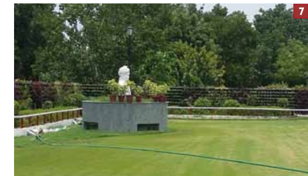
Ventilators of underground parking used as platform for mounting sculpture
