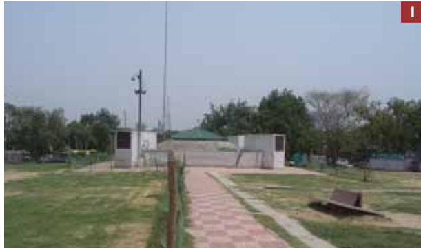
Skylights to render diffused light to the market below
