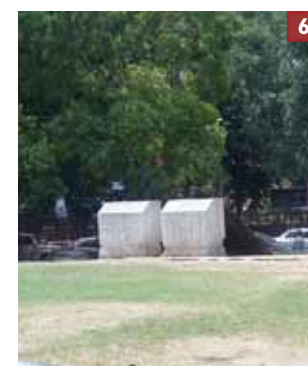
Toilets (below) ventilator
