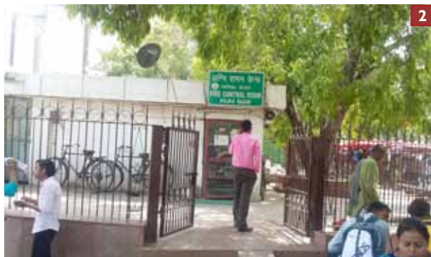
Fire Control Room, accessible from the footpath level, gated and fenced
