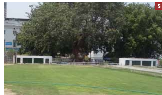
Ventilators of underground parking exist as pop-up structures onto the area above it
