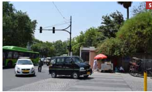
Shows the edge of the site from Outer circle to Panchkuian Road Source: DUAC, 2017 (photograph), New Delhi
