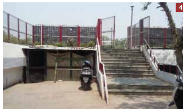
Entrance to the area above Palika parking from the road between Palika parking and the shopping complex and near to the Outer circle
