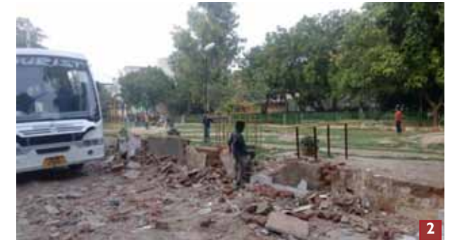
Dilapidated condition of the park adjacent to green belt
