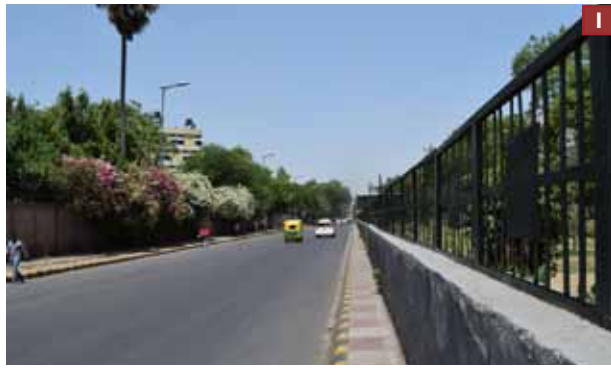
Shows the edge of the site as seen from the Panchkuian Road Source: DUAC, 2017 (photograph), New Delhi
