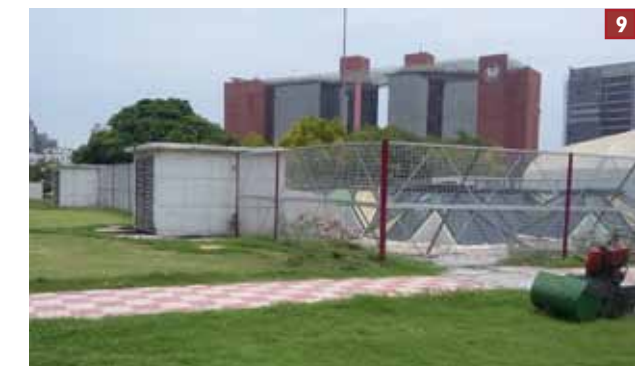
Skylights for underground parking
