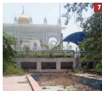
Ventilators of underground car park open onto the site
