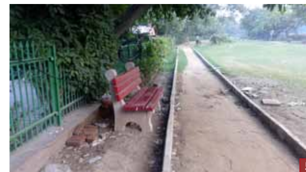
Lack of appropriate pathway for the users
